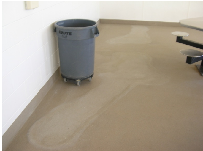
Discolored Sections of New Floor
