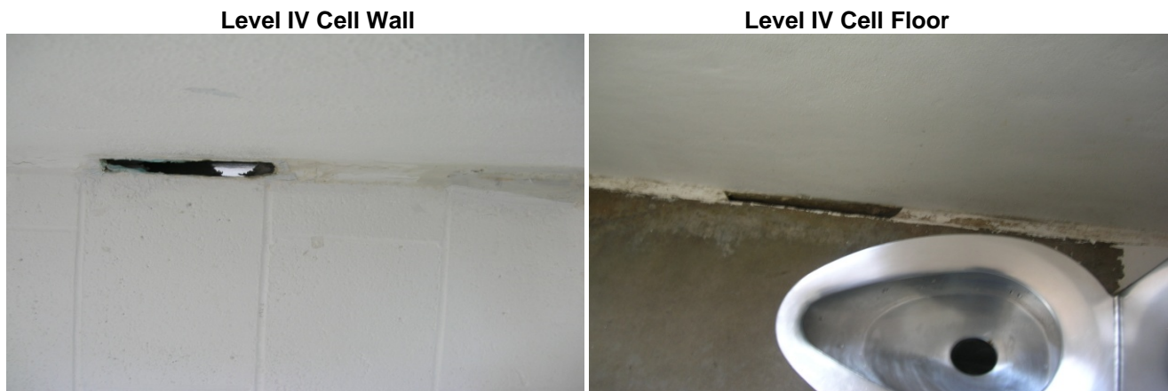
Figure 6. Holes in SNMCF Level IV Facilities
