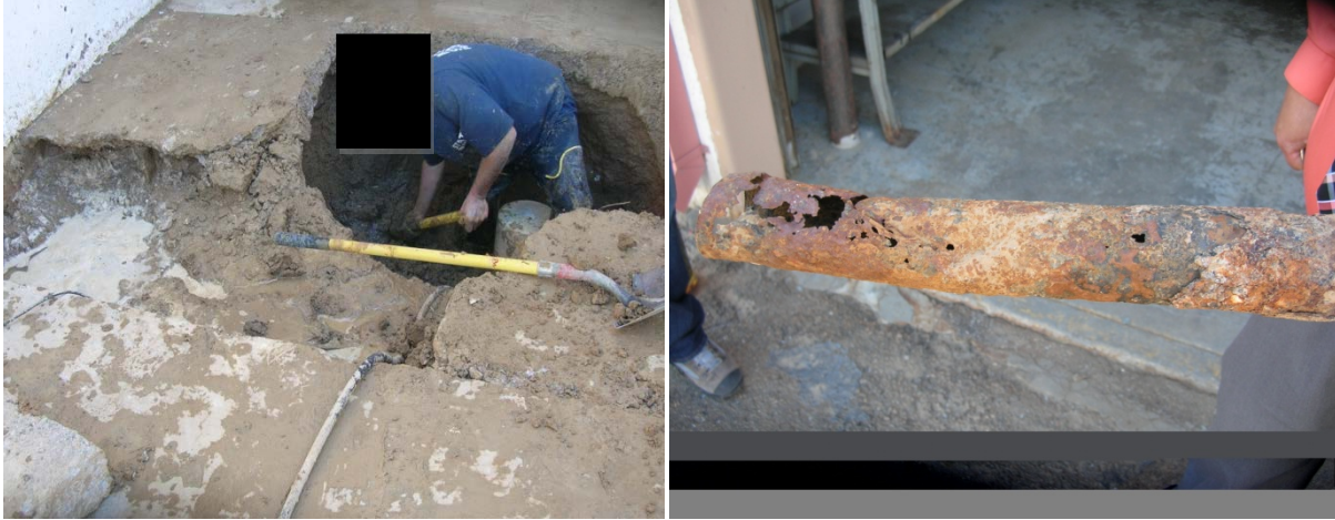
Figure 1. Water Leak Repair and Corroded Pipe at WNMCF
