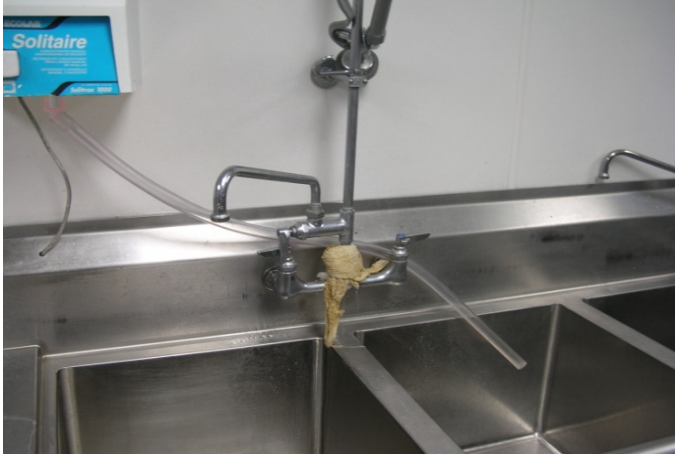
Leaking Sink
